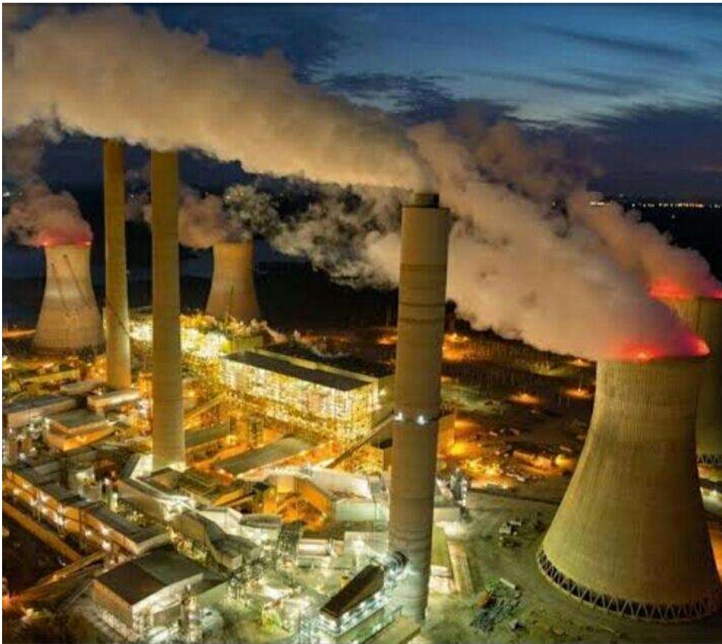
Fig 3. Coal fired power plant
